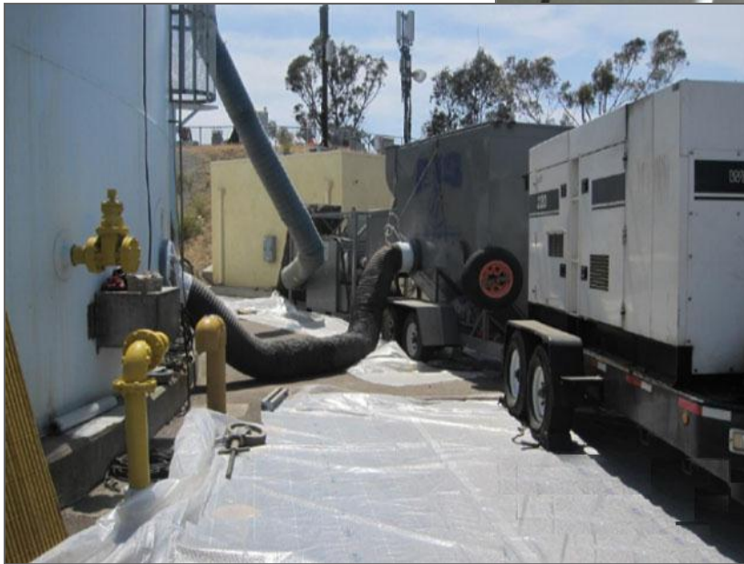
832-2 Ventilation and interior blasting equipment
