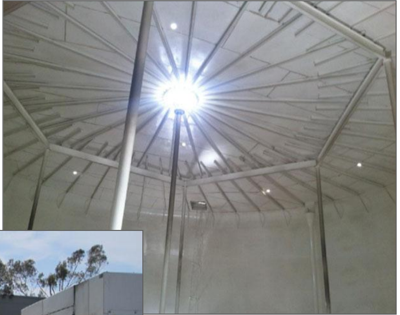
803-3 Reservoir interior coating progress
